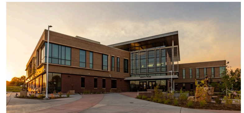
Larimer County Campus Fort Collins, CO
