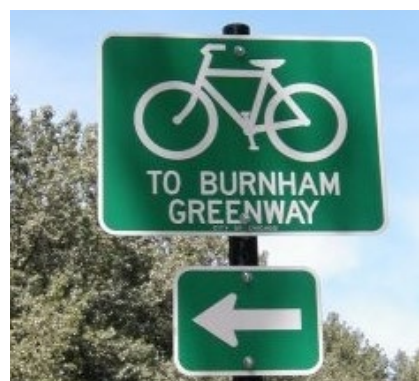
Directional arrows may be added to a bike route sign to clarify the need for a turn movement, Chicago, IL.
