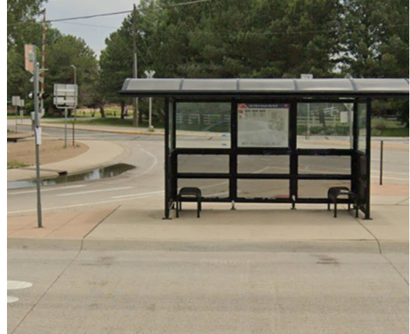
Figure 7. Existing bus stop at Niwot Park-n-Ride heading northeast.
